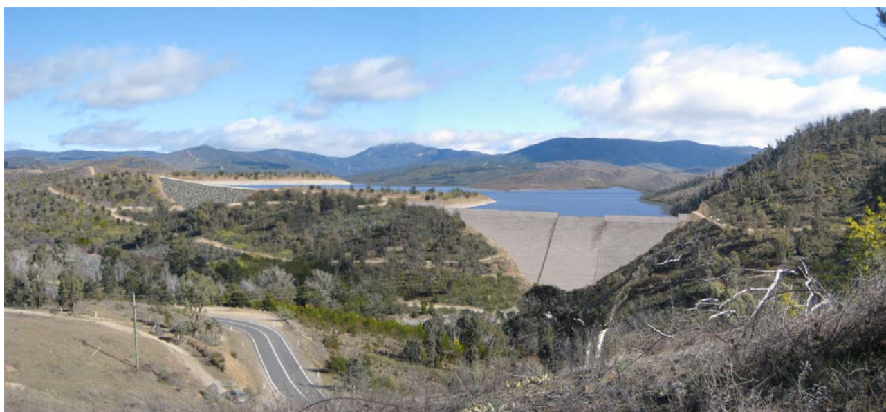
Figure 12 Artist's impression of the Enlarged Cotter Dam after completion and when full
