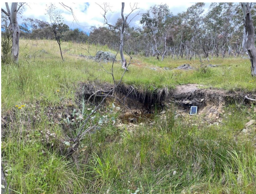
Figure 30: Erosion point 13; as observed during baseline surveys in 2012 (top) and in 2022 (bottom).
