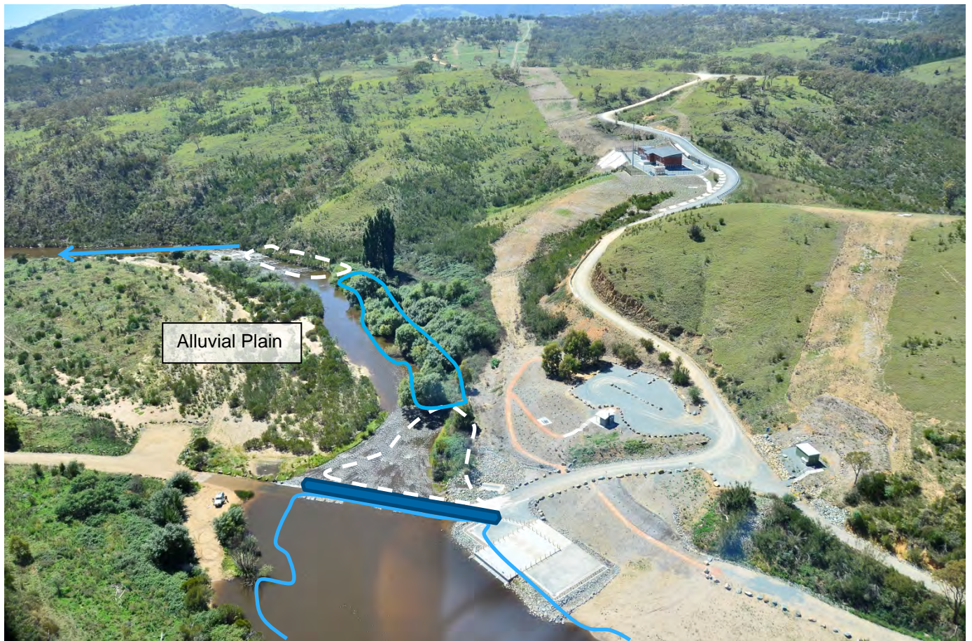
Figure 18 - Angle Crossing Channel Units 10/3/2013
