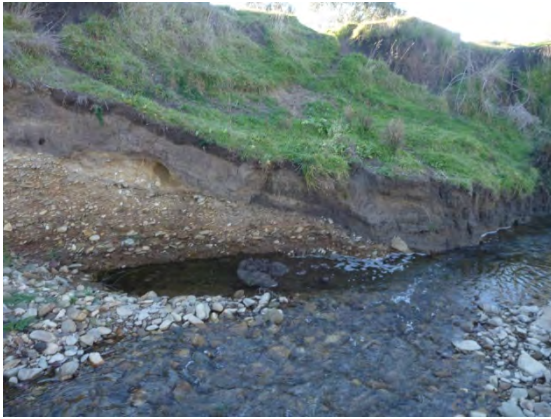
Photo 4 - Erosion potential area downstream of Pool 5 control in June 2014 (left) and September 2014 (right) –new erosion above gravel layer in embankment
