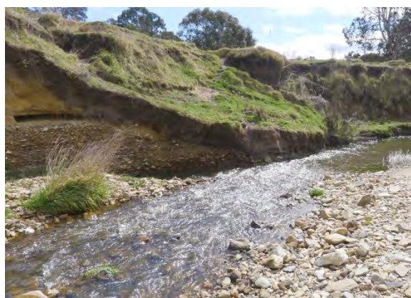
Photo 4 - Erosion potential area downstream of Pool 5 control in June 2014 (left) and September 2014 (right) –new erosion above gravel layer in embankment
