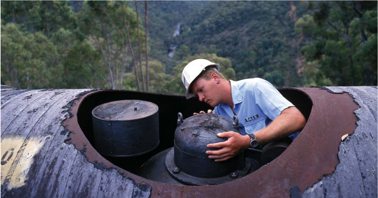
Essential pipeline maintenance
