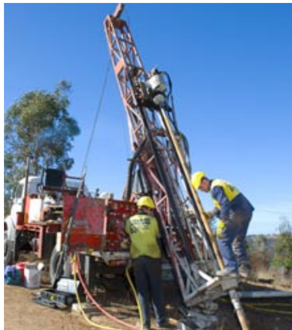
PRELIMINARY WORK FOR THE ENLARGED COTTER DAM.
