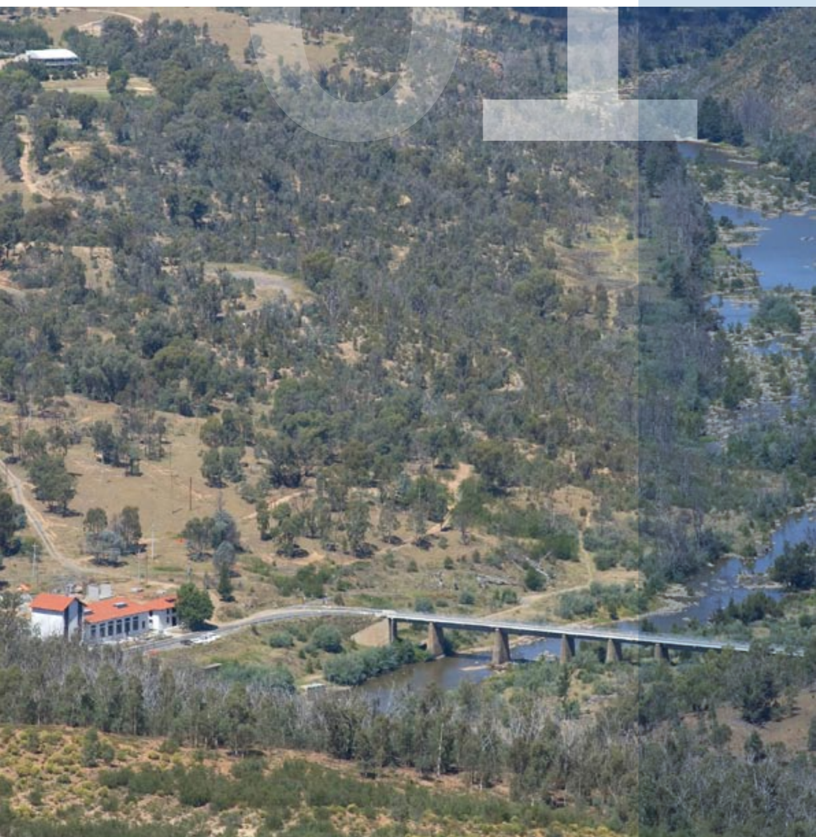
THE COTTER PUMPING STATION.
