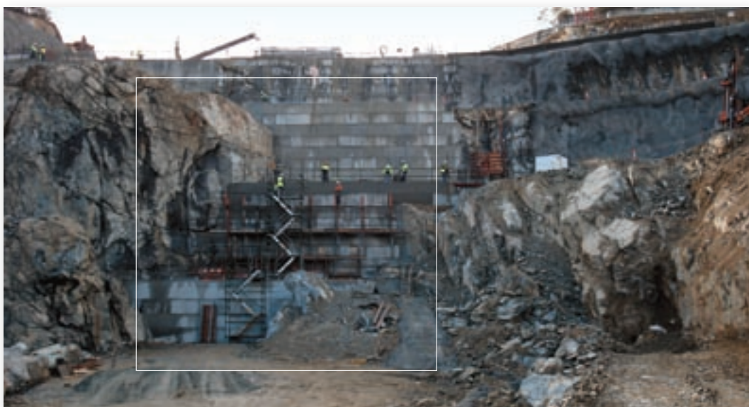
Upgrading Googong Dam Spillway
