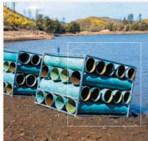
Protecting endangered fish species: Provision of artificial fish habitat as part of the Enlarged Cotter Dam project.
