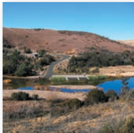
Artist impression of low lift pump station on the Murrumbidgee River which is part of the Murrumbidgee to Googong Water Transfer project
