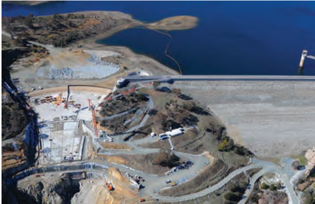
Construction at Googong Dam Spillway
