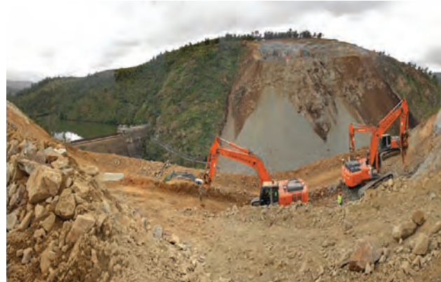
Enlarging the Cotter Dam
