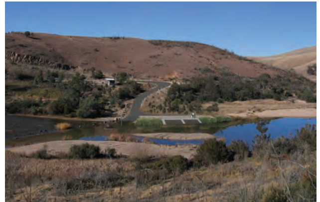
Artist's impression of low lift pump station for Murrumbidgee to Googong Water Transfer
