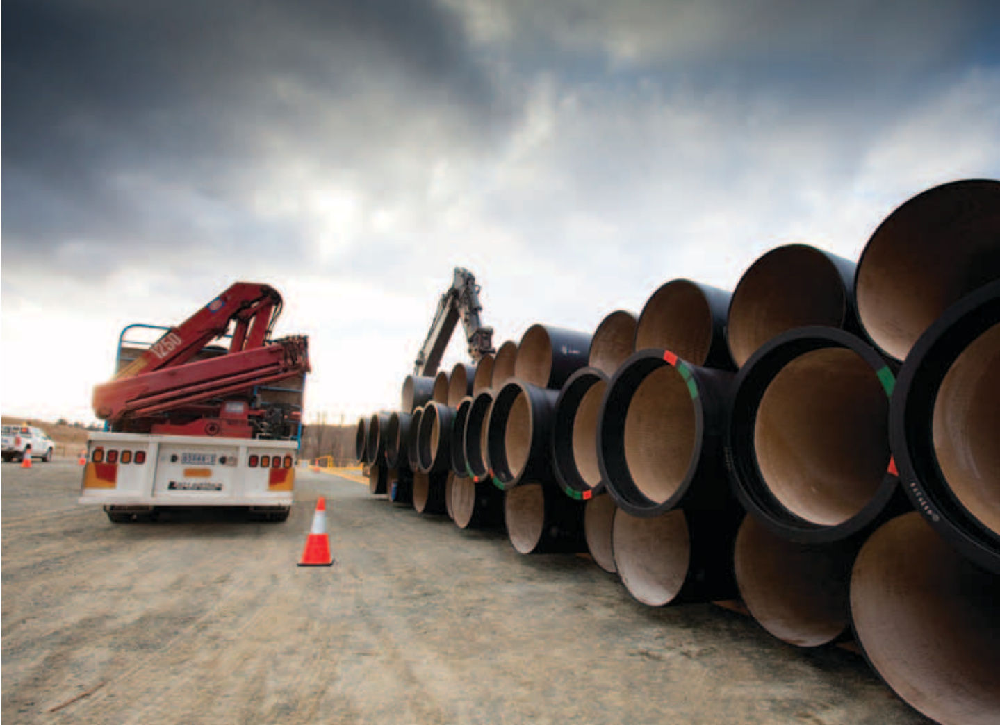
Pipes for the Murrumbidgee to Googong Water Transfer.
