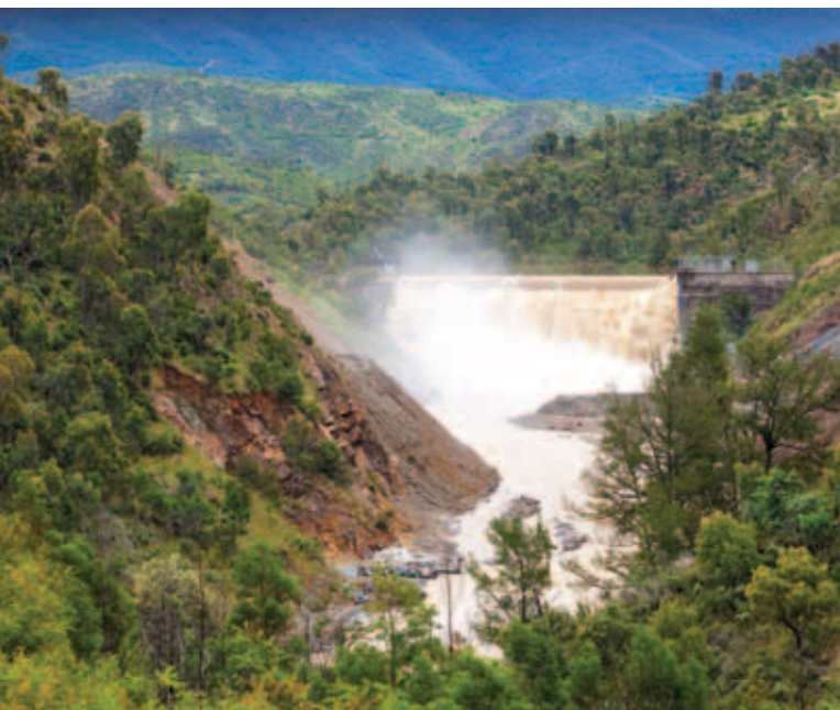
The existing Cotter Dam overflows in December 2010 following heavy rainfall.
