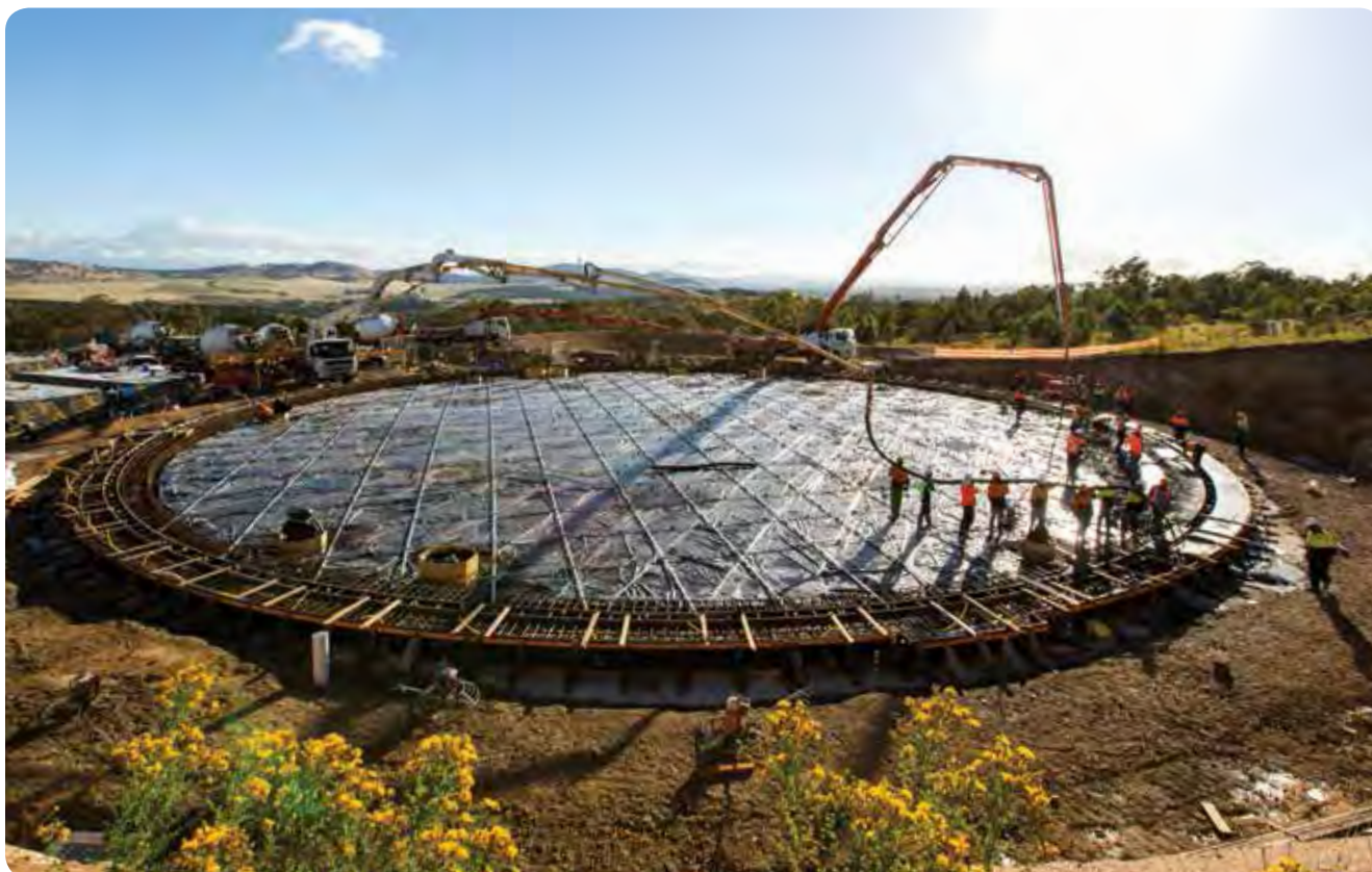
Molonglo Valley Reservoir (construction)
