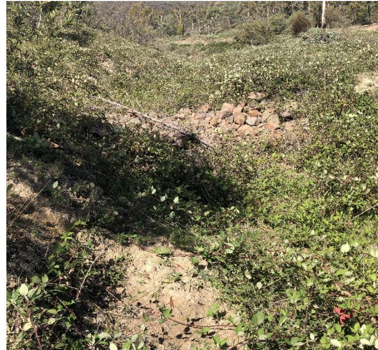
Site MZ4a looking downstream along gully obscured by blackberry
