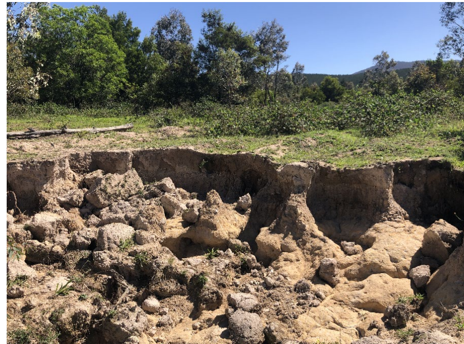
Site MZ4b: looking upstream at head cut within drainage depression
