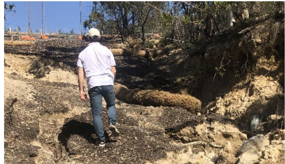
Site MZ1a looking upstream from 50 south of East West Break crossing
