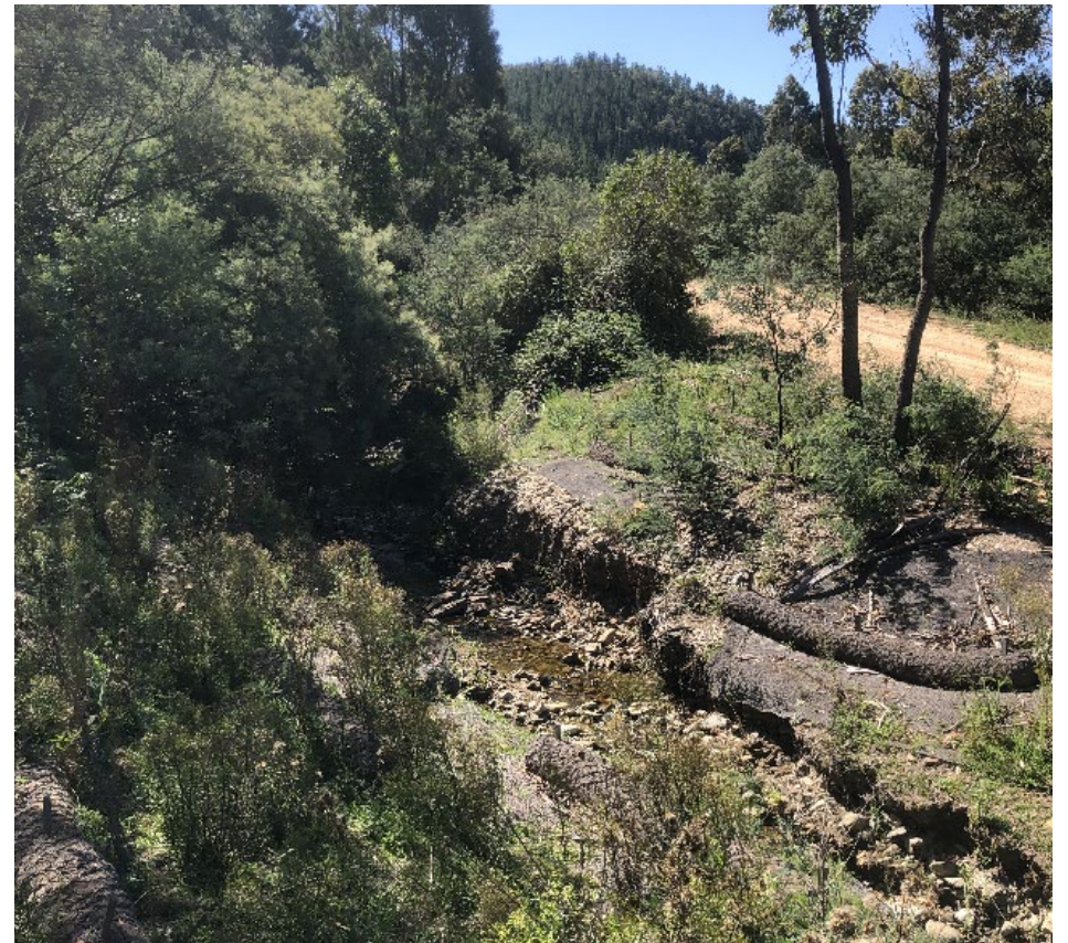
Site MZ6: Looking upstream Lees Creek, with washed out rehabilitation works in foreground
