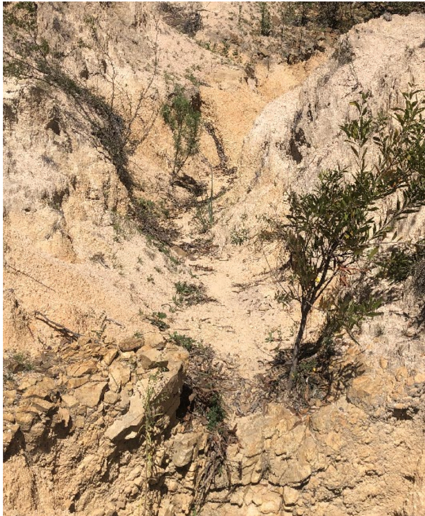
Site MZ2 looking upstream towards Pierces Creek Rd
