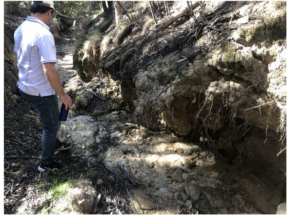
Site MZ5. Fluvial scour contributing to widening of the channel
