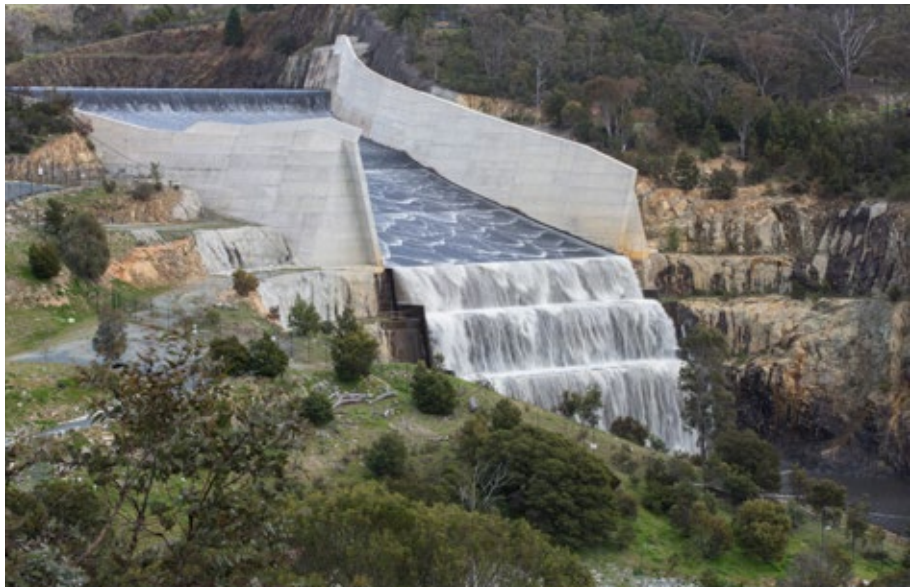
Googong Dam spilling
