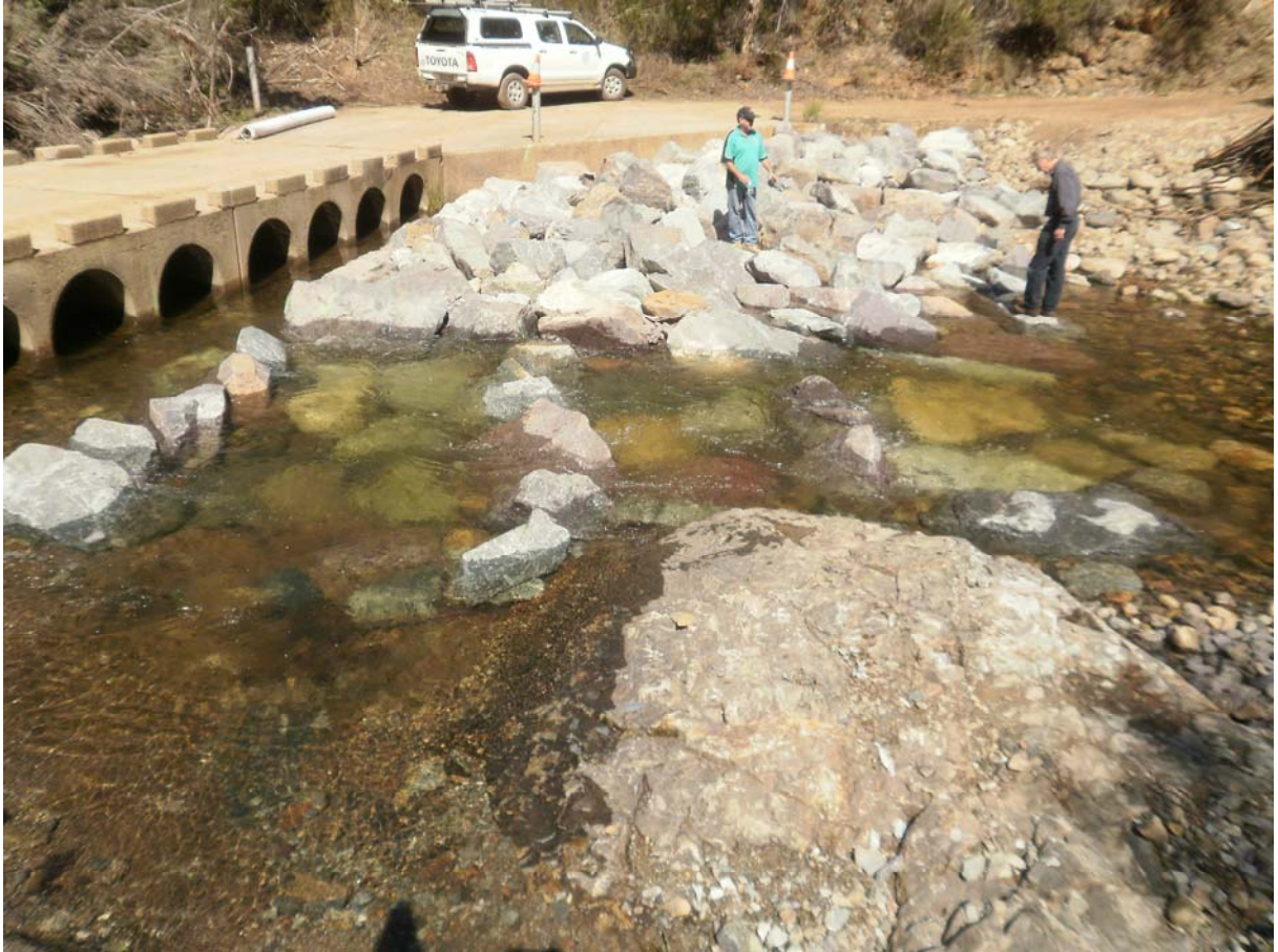
Plate 7 - Completed fishway under low flow conditions
