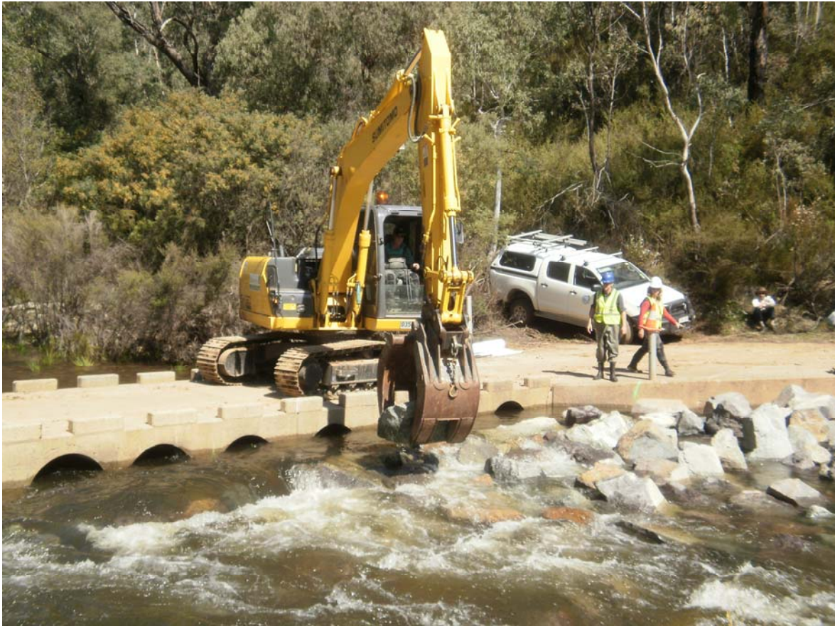
Plate 6 - Fishway construction under high flow conditions
