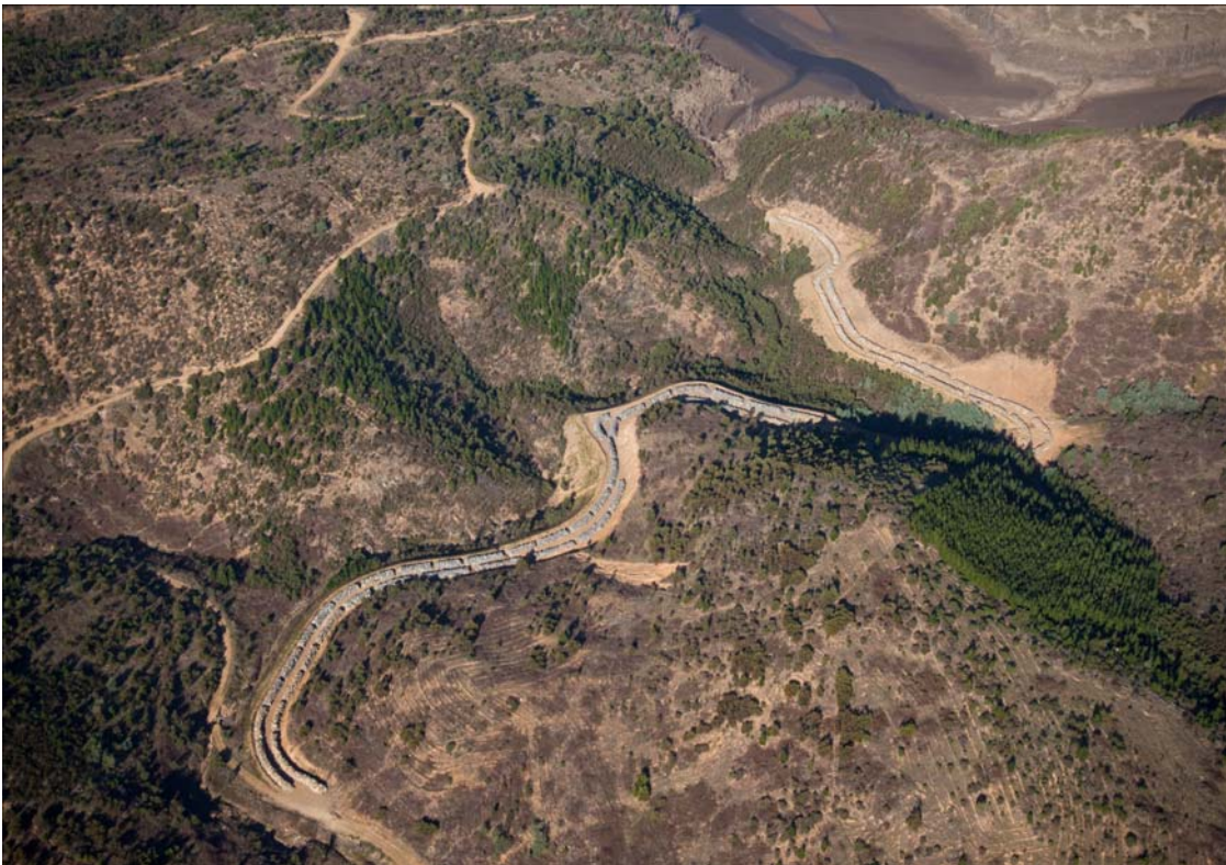
Plate 3 - View of rock reefs constructed on Priors Road
