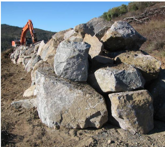
Plate 1 - Construction of rock reef habitat on Gully Road
