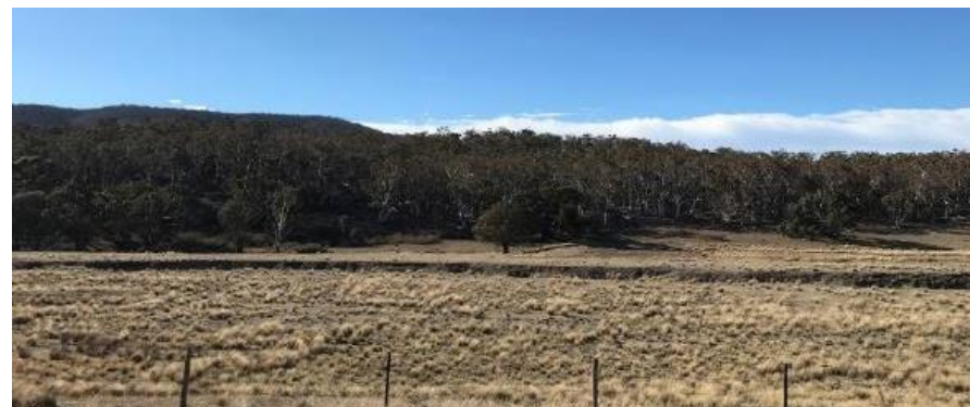
Site MZ5b looking from Burra road towards Cassidy's Creek. Note eroding right bank running through centre of picture. Estimates based on banks upstream and from lidar puts this bank at 3-5m vertical.
