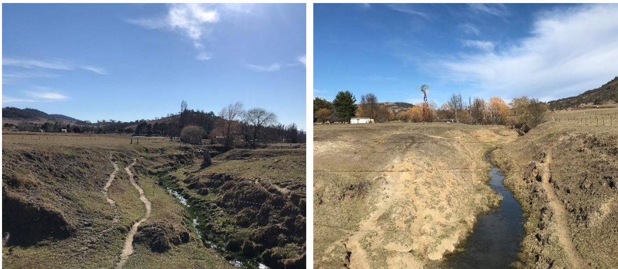
Figure 12. Example of stock impacted waterways within Googong catchment. Note informal tracks along banks
