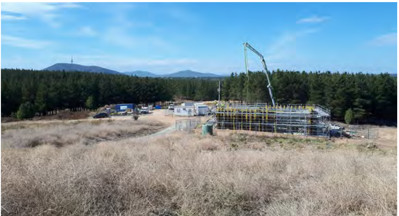
Construction of fanhouse
