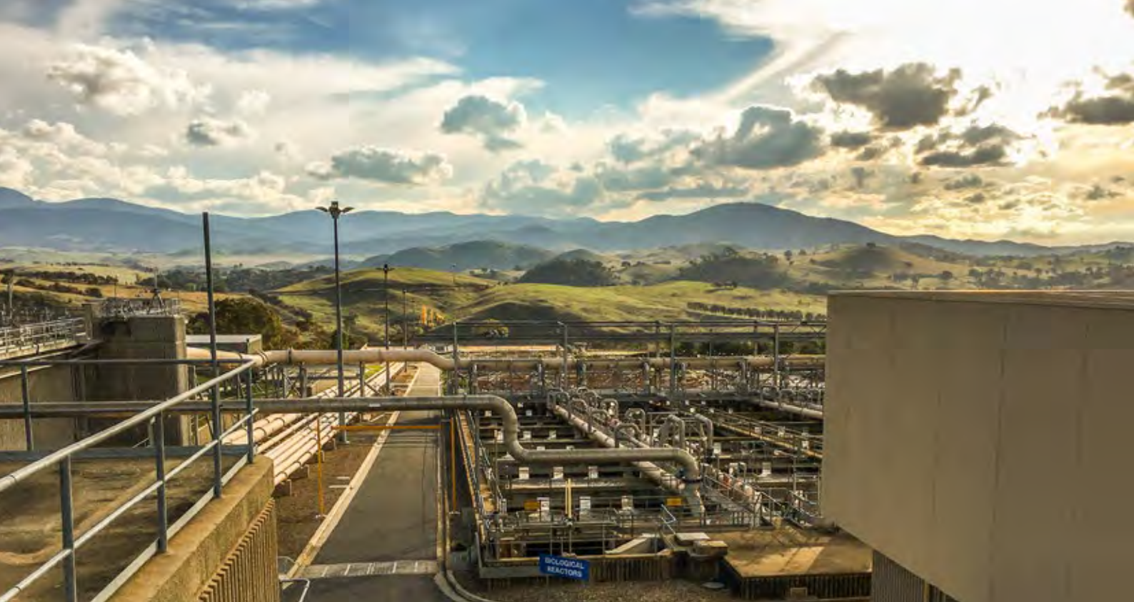
Lower Molonglo Water Quality Control Centre
