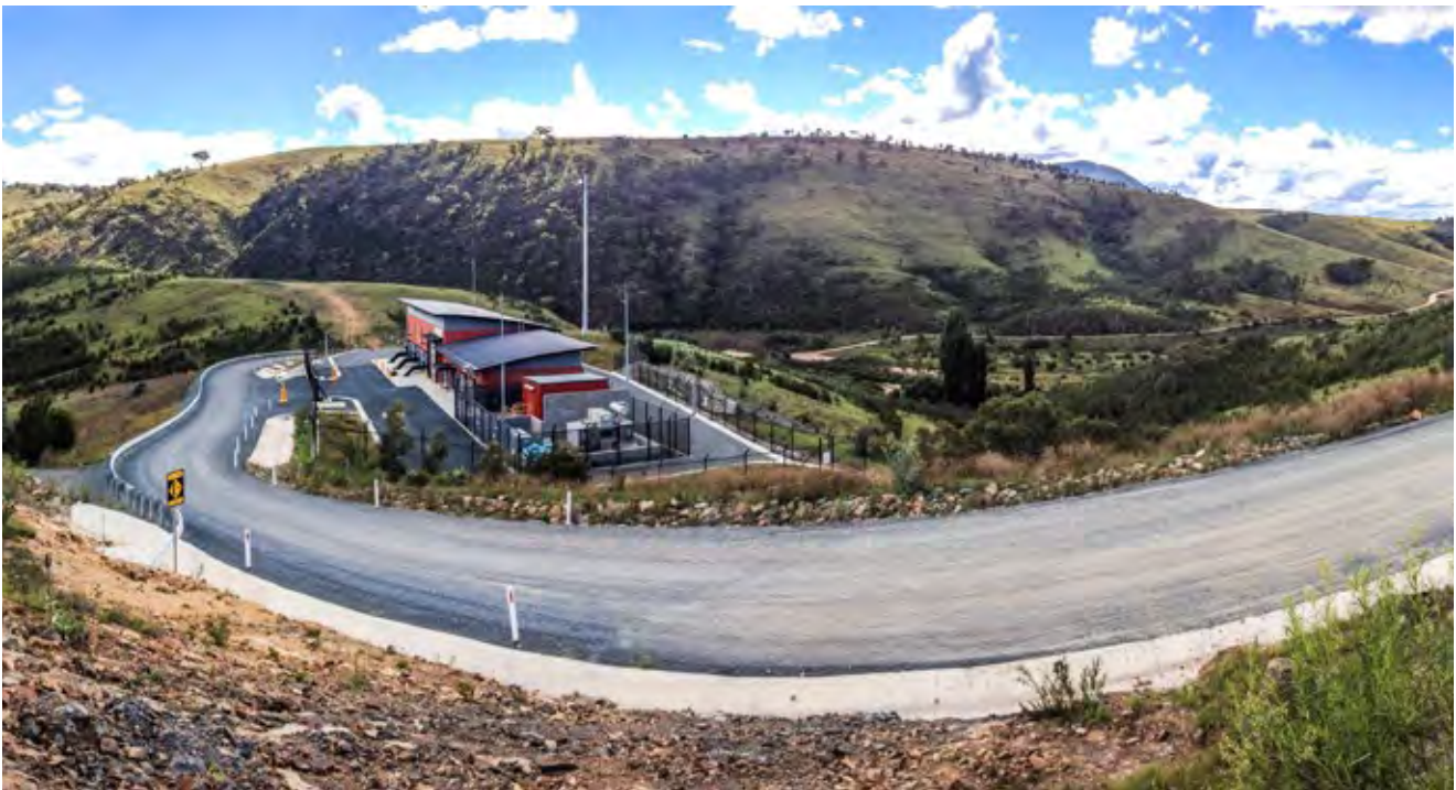
Angle Crossing High Lift Pump Station M2G
