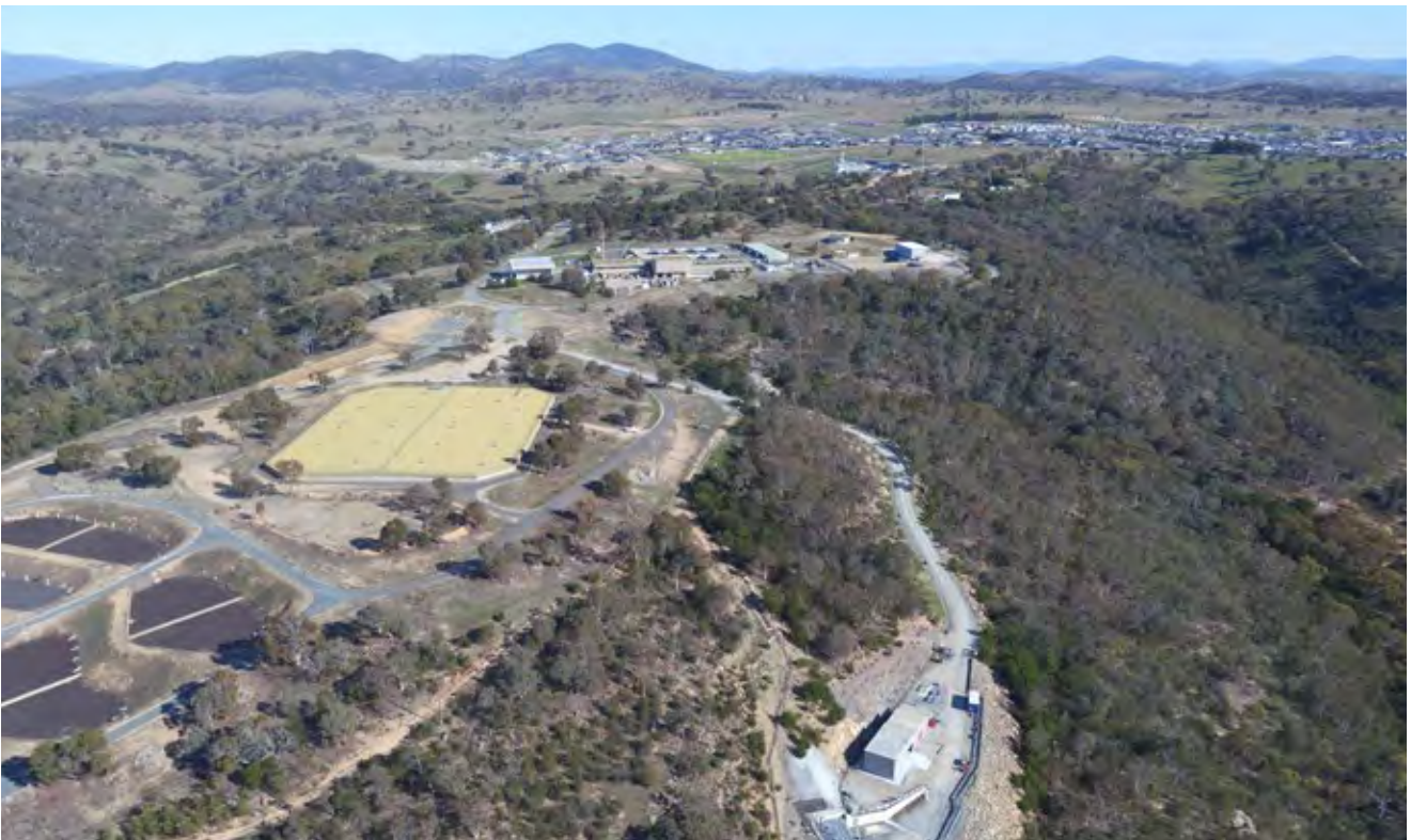
Googong Treatment Plant
