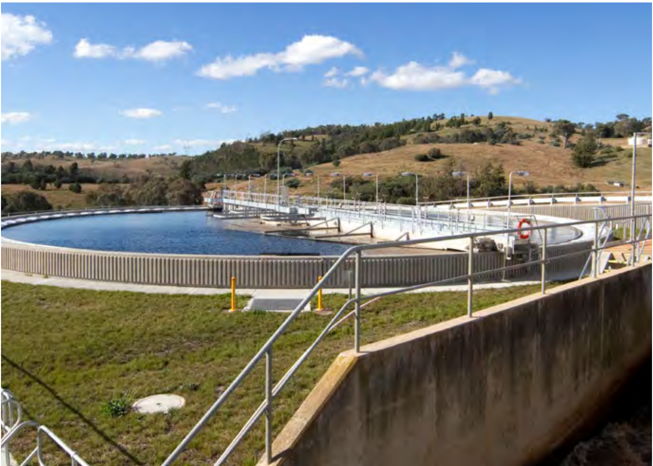
Lower Molonglo Water Quality Control Centre - Secondary Clarifier
