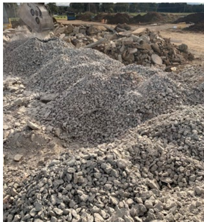
^ Crushing operation underway at Fyshwick
