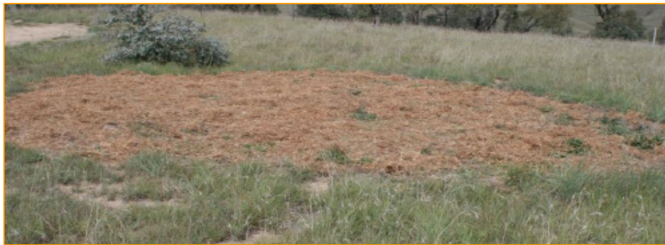
Figure 5.3 Typical application of Themeda mulch as part of rehabilitation activities on the M2G project.
