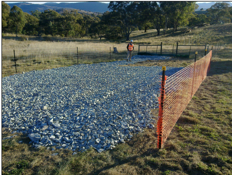
Figure 2.2 Typical weed wash down bay.
