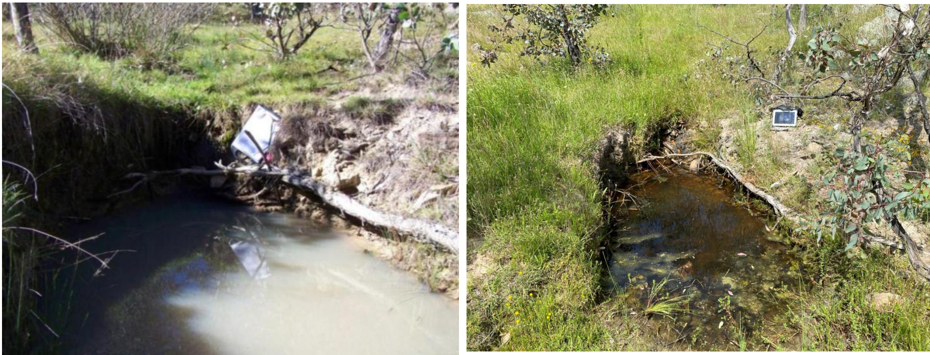
Figure 30: Erosion point 4; as observed during baseline surveys in 2012 (left) and in 2020 (right)
