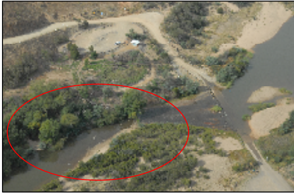
Mur 19. Downstream Angle Crossing
