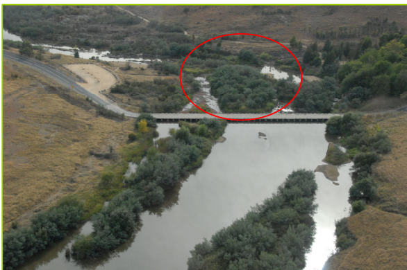
Mur 23. Point Hut Crossing
