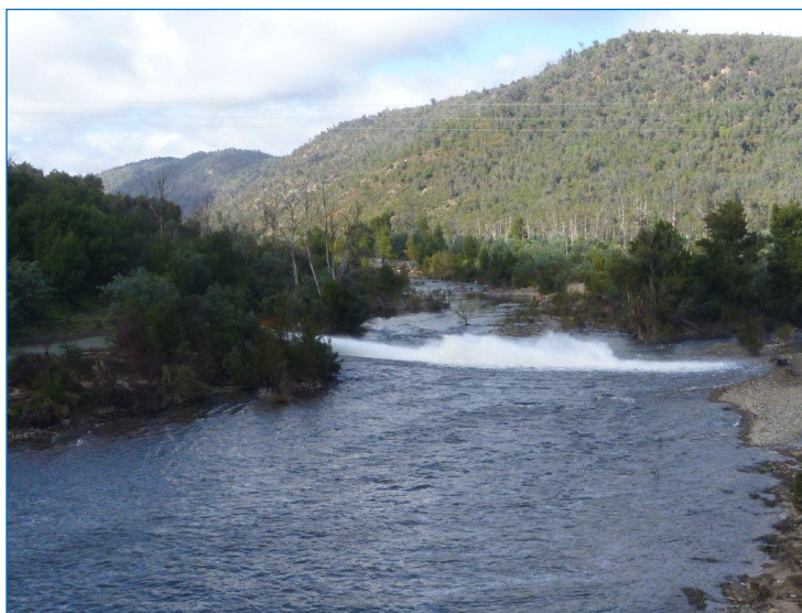
Plate 5. Bendora Main Scour during the first week of May
