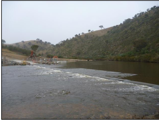
MUR 19 Looking across at the construction
