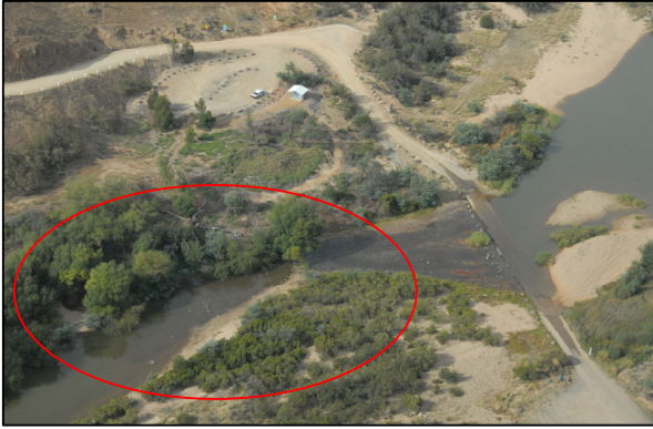
Mur 19. Downstream Angle Crossing
