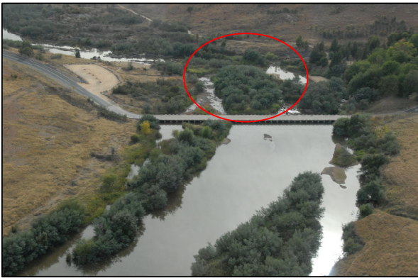
Mur 23. Point Hut Crossing
