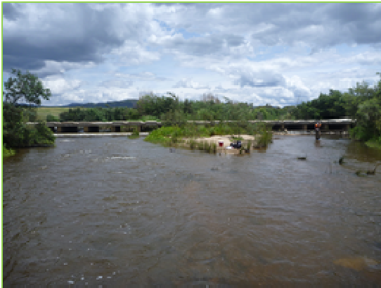
Mur 23. Point Hut Crossing
