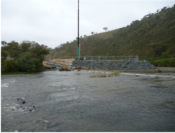
MUR 19 Downstream of Angle Crossing looking up to the coffer dam
