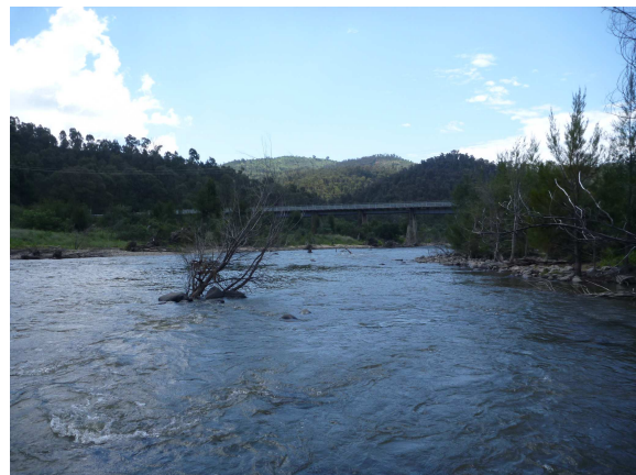
MUR 28 Looking downstream towards the Road Cotter Bridge
