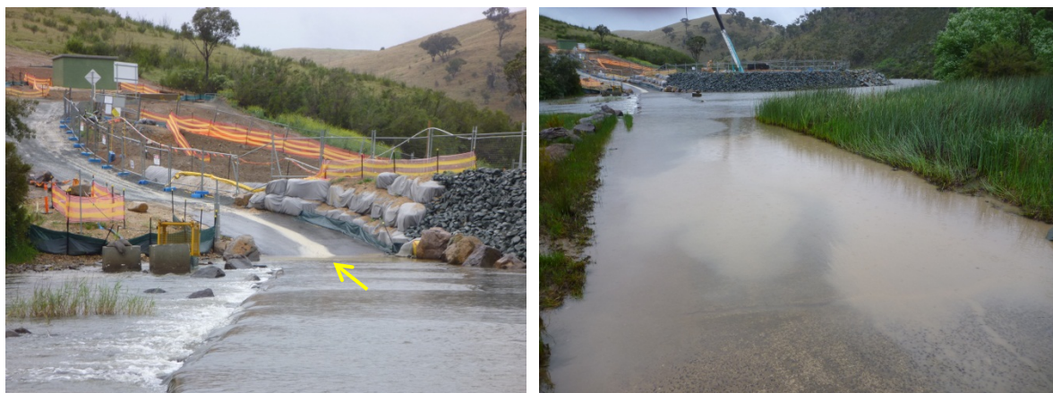
Plate 4.1 - Angle Crossing, showing turbid runoff from the right hand (indicated by the arrow) and from the left hand side
