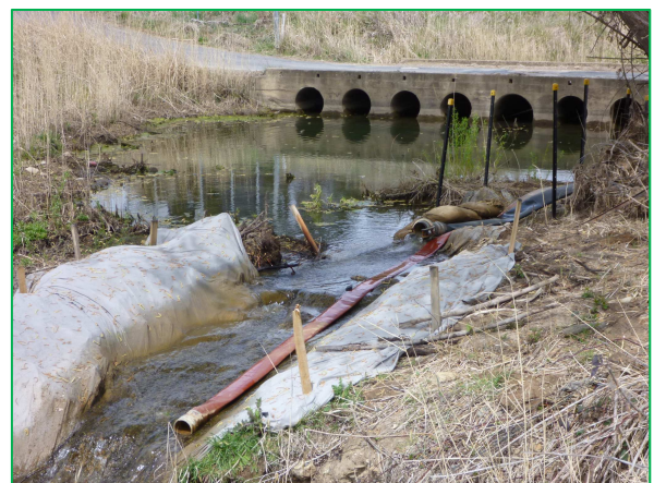
Plate 1. Looking downstream Williamsdale Bridge (left) and creek water being diverted downstream of Williamsdale Bridge during construction
