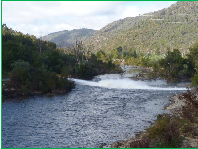
Plate 4. Bendora scour valve operational near MUR 28
