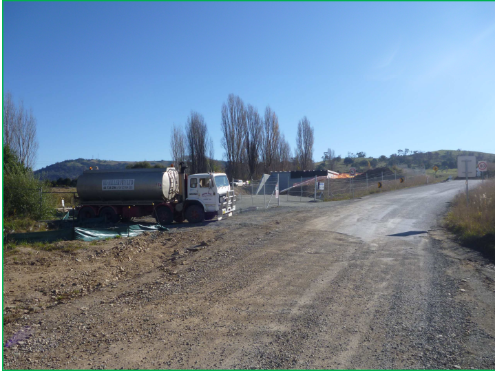
Plate 2. M2G construction site on the western side of Williamsdale Road Bridge
