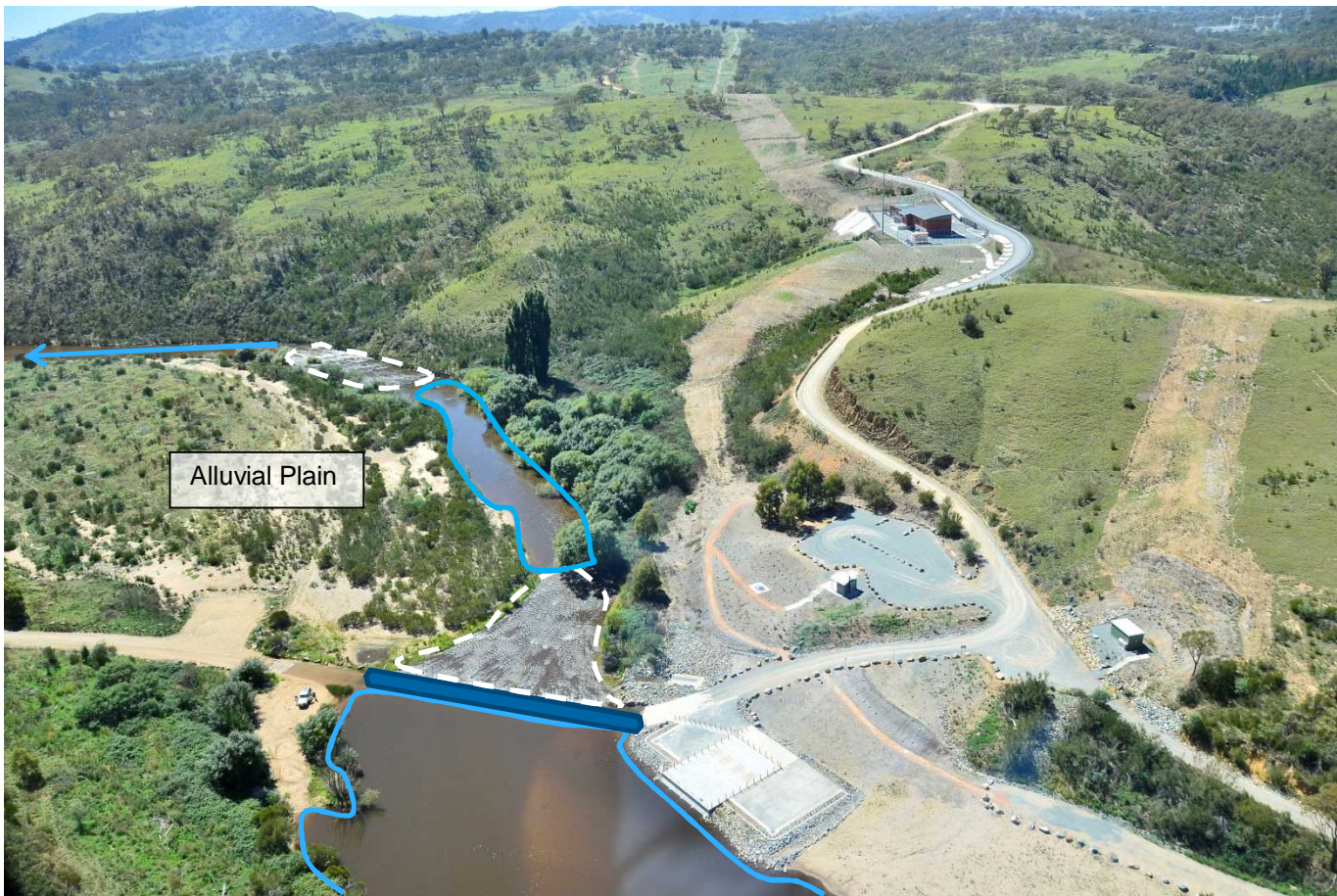
Figure 10 - Angle Crossing Channel Units 10/3/2013
