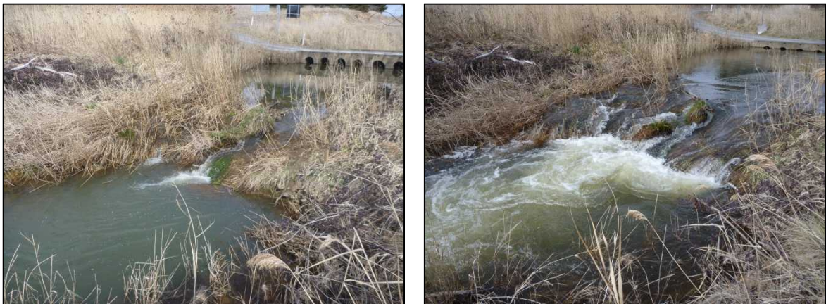
Plate 1. Step with moderate adjustment potential immediately downstream of Williamsdale Road, left at <5 ML/d, right at 100 ML/d
