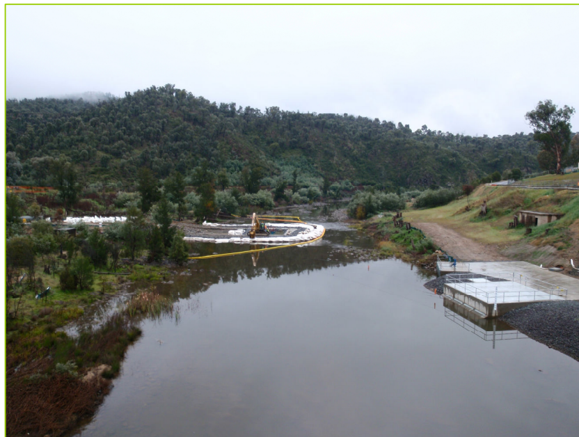
Plate 1. The Murrumbidgee River from the Cotter Road Bridge. Top: looking upstream towards the Cotter River confluence. Bottom: looking downstream with the MPS pump intake on the right and the Coffey dam wall on the left hand side*. At the time these photographs were taken (26/05/2010), the mean daily flow at Mount MacDonald (410738) was 36.7 ML/d.
