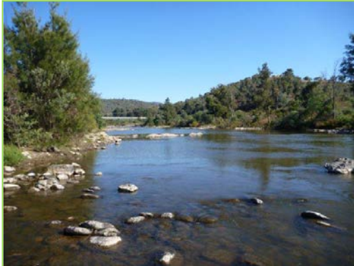
MUR 935. Looking upstream to Cotter Road Bridge
