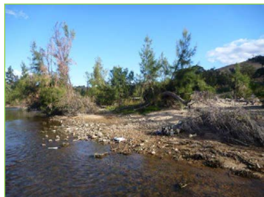
MUR 29. Flood damage to riparian zone
