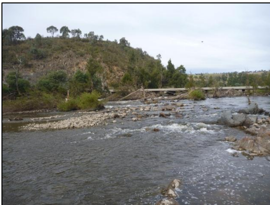
MUR 29 Looking upstream towards Uriarra Rd.
