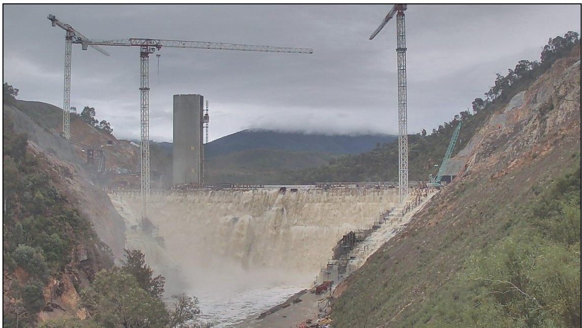
Plate 3. Enlarged Cotter Dam construction during March event, 2/5/2012 (Source: www.actew.com.au)
