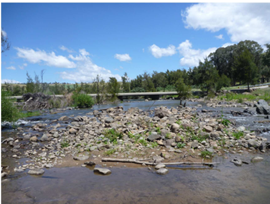
MUR 29 Looking upstream towards Uriarra Rd
