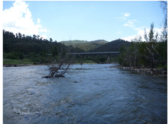
MUR 28 Looking downstream towards Cotter Bridge
