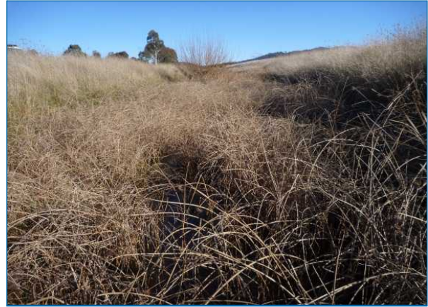
BUR 1c Encroachment through the riffle habitat
