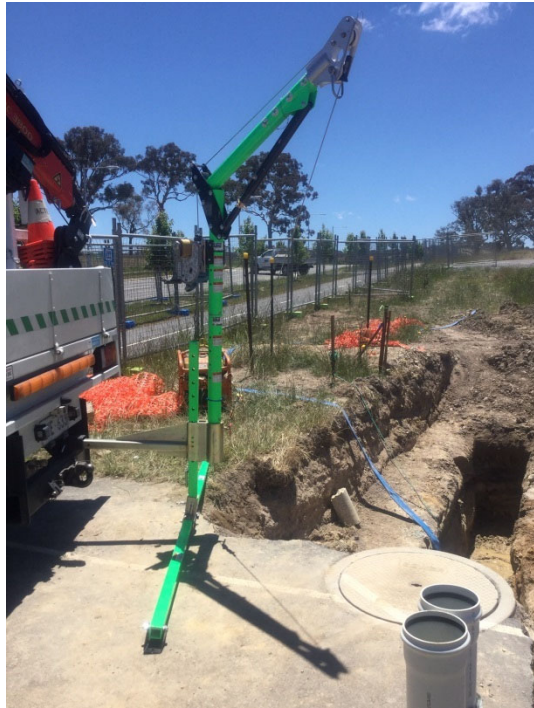
Fig. 5.7.4.2.1 A tow-bar mounted davit being set-up over a maintenance hole
