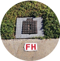
In ground valve or hydrant
