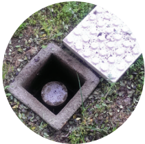
Sewer riser or inspection shaft
