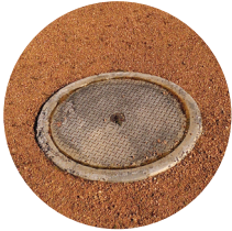
Sewer maintenance hole
