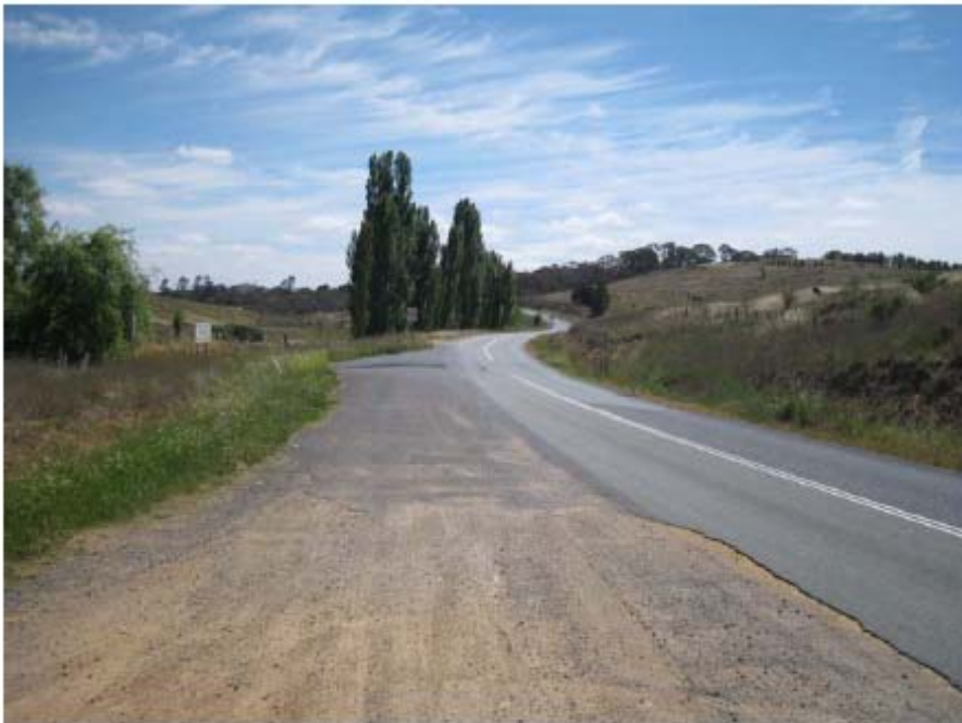
Photo 15: Burra Road northbound approaching Williamsdale Road intersection
