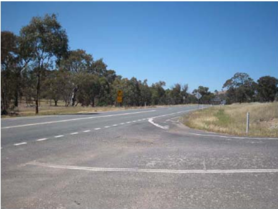
Photo 6: Angle Crossing Road/ Monaro Highway intersection looking south
