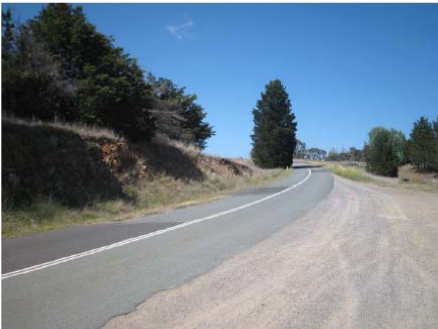
Photo 16: Burra Road southbound from Williamsdale Road
