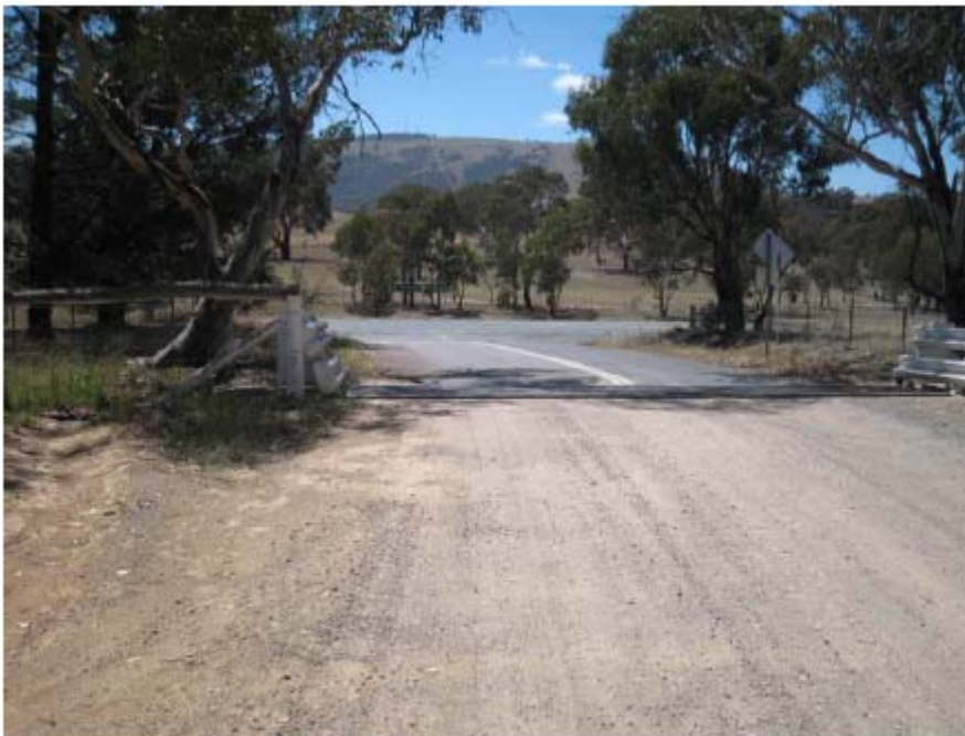
Photo 4: Angle Crossing Road approaching Monaro Highway
