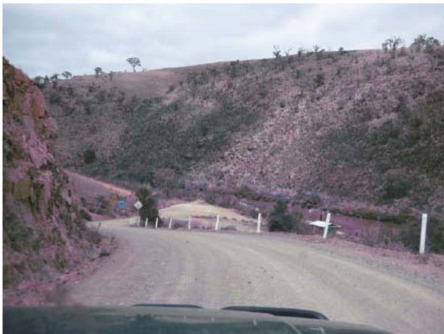
Photo 2: Angle Crossing Road approaching Causeway
