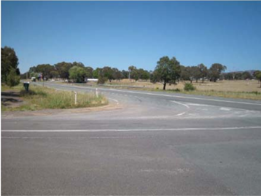
Photo 7: Williamsdale/ Monaro Highway intersection looking south
