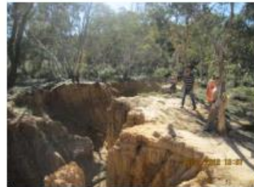
Headward erosion at tributary confluence with Buchan Creek
