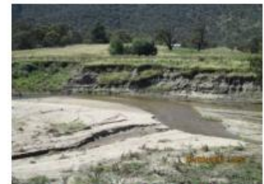
Bank erosion along the Naas River
