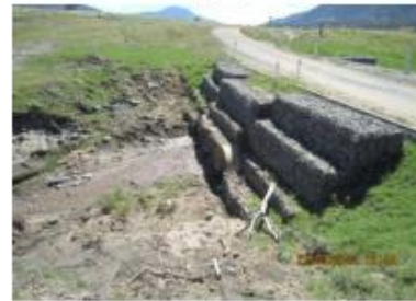
Rock gabion headwalls on Naas Road
