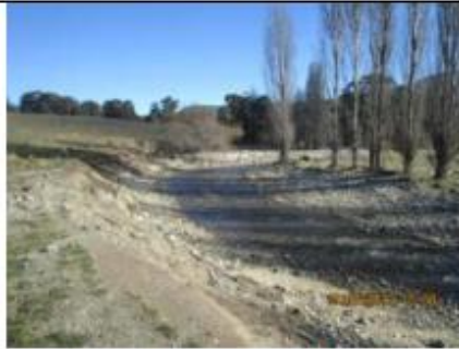
Sedimentation downstream of the bridge
