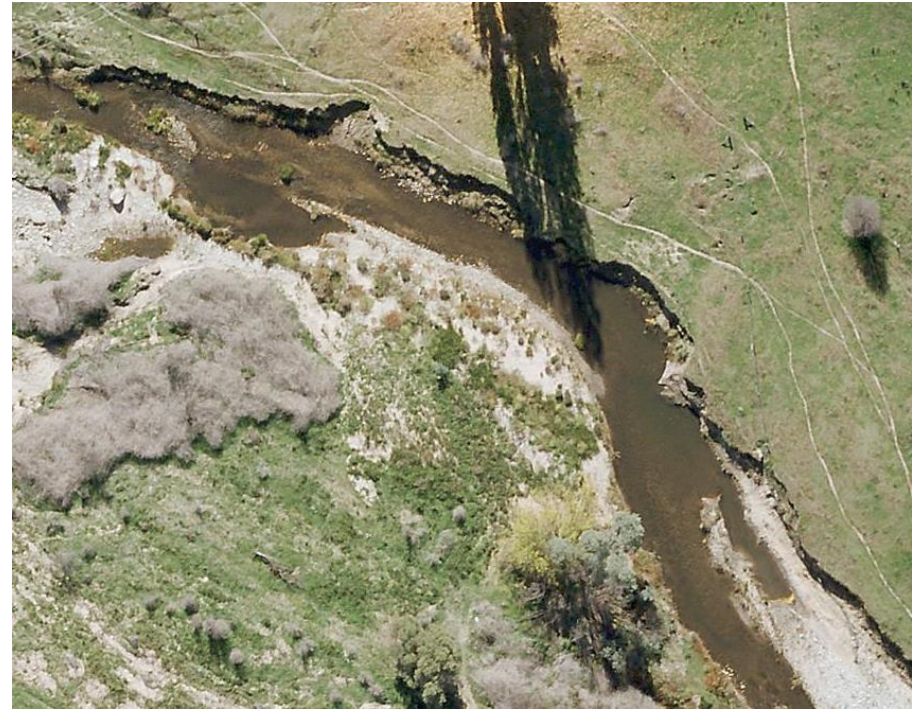
2017 aerial image of erosion requiring further investigation identified upstream from site
