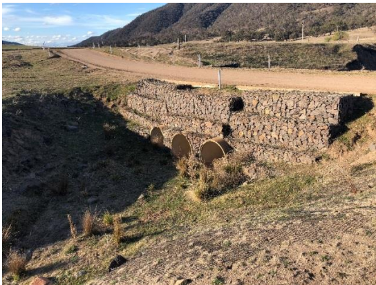
Rock gabion headwalls on Naas Road
