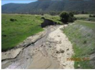
Large areas of fine sediment deposition
