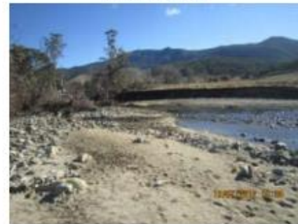
Major bank erosion
