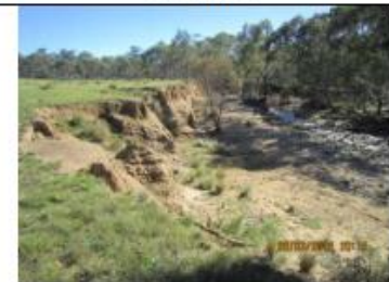
Bank erosion Buchan Creek
