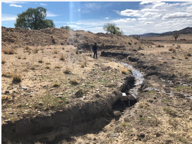
New low flow channel slowly moving its way upstream
