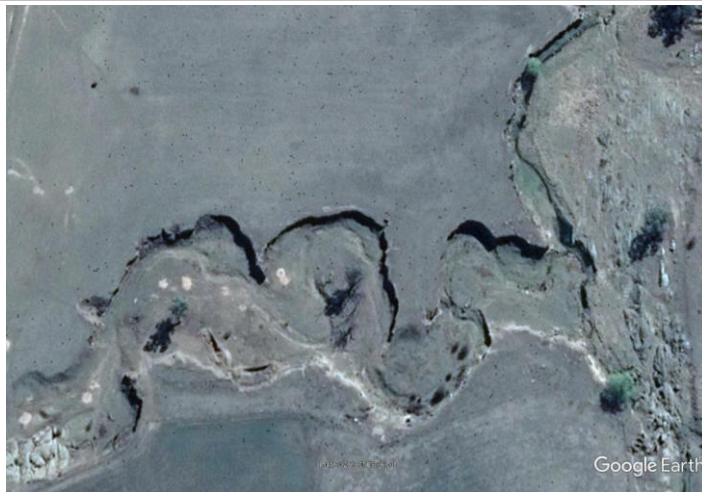
September 2018 aerial image of bank erosion in Bakersdale Creek and Murrumbucca Creek (down-stream of the confluence)
