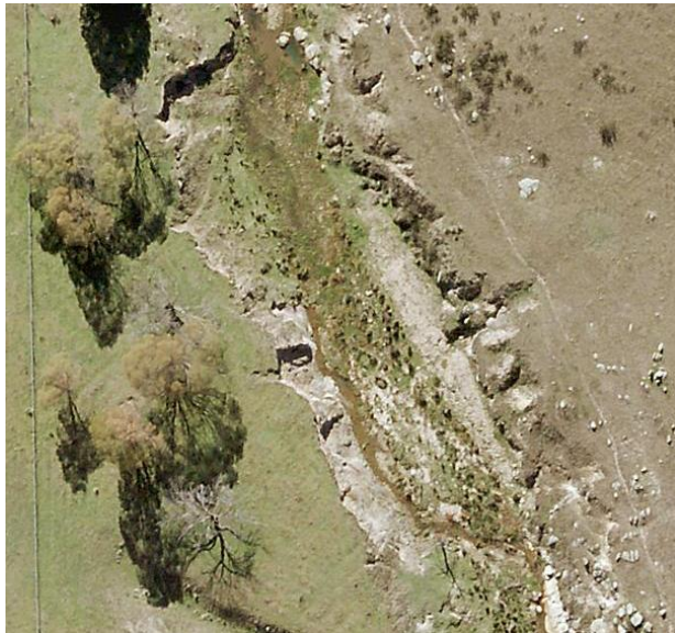
2017 aerial of bank erosion in Spring Station Creek upstream of the confluence with the gully
