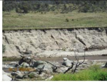
Widespread bank erosion along Naas River
