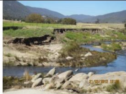
Further bank erosion downstream
