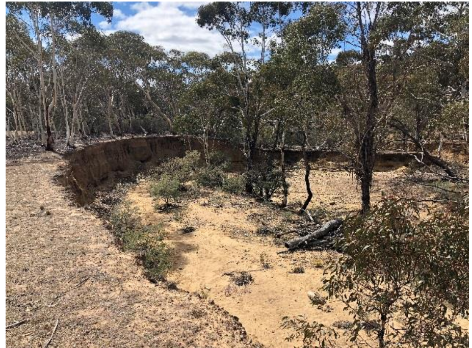
Bank erosion Buchan Creek
