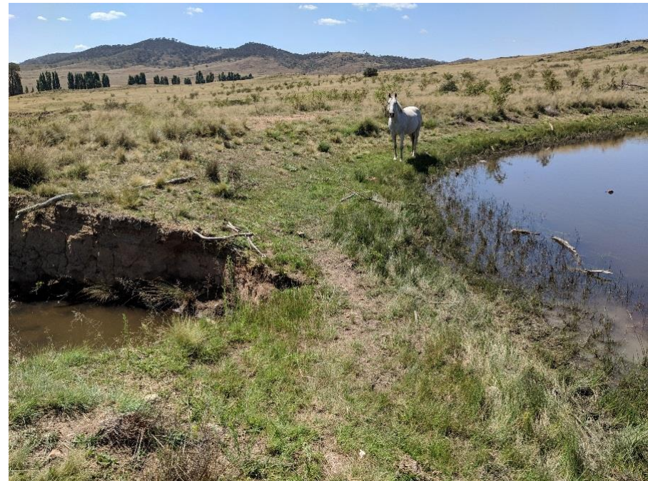
Head cut migrating through the embankment
