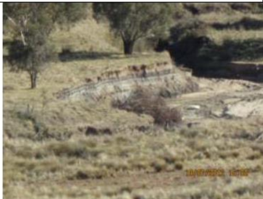
Bank erosion at the confluence
