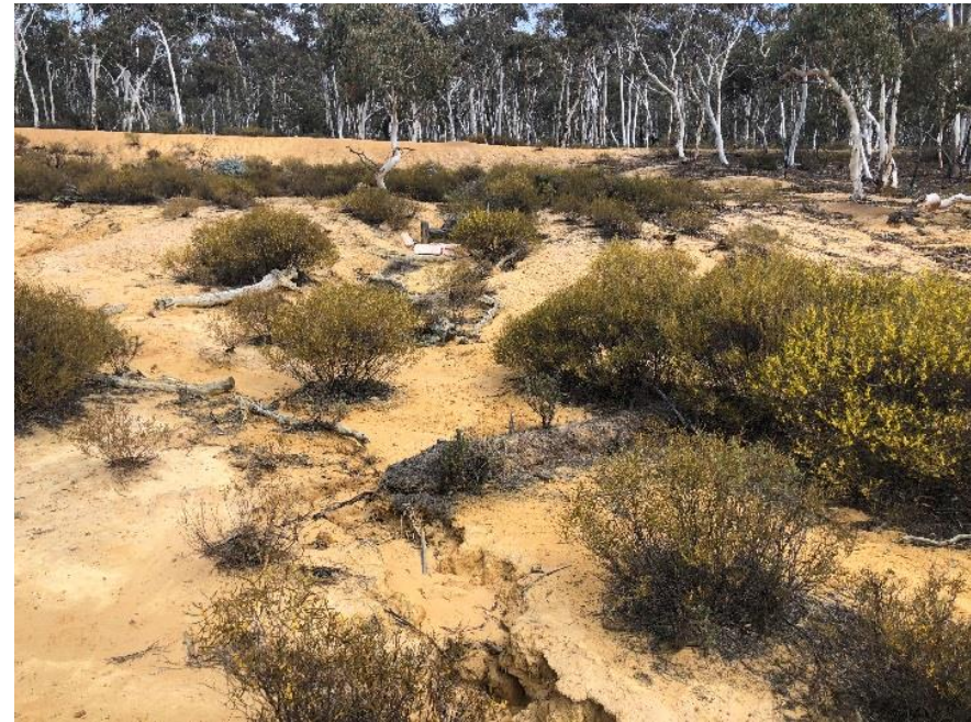
Coir logs on slope washed away with small gullies forming
