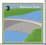
This is the smallest Dam along the Cotter River and is located between the Corin and Cotter Dams. This curved structured holds 11.4 billion litres when full (equivalent to 4,560 Olympic sized swimming pools). We use gravity to send water to Mount Stromlo, from Bendora, through a 20 km pipe.
