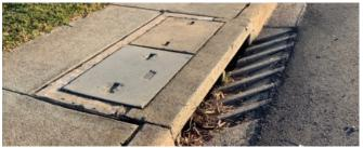
There are also drain pipes outside your house that collect rainfall runoff from roofs, driveways, footpaths, carparks, and roads that connect to the storm water drainage network. These drains are separate to the sewage system, taking rainfall from gutters on our roads, flowing into local waterways, lakes and rivers.
