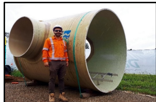
Each GRP precast manhole has a circumference of 2.5 metres!
