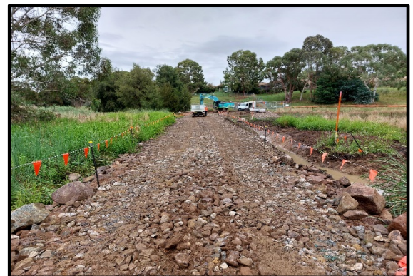
Work on the pipeline bridge across Ginninderra Creek will commence shortly
