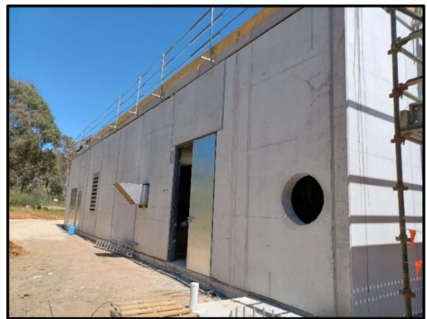
The external walls comprise precast concrete panels.
