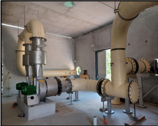
Ductwork as part of the mechanical fit out inside an OCU.
