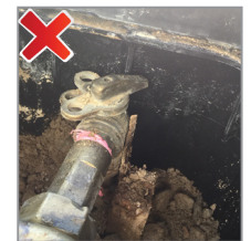
No clearance for Ball valve
