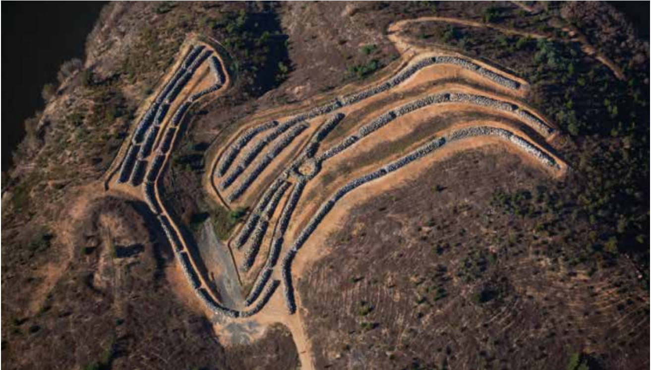
Satellite image of the rock reef artificial habitat constructed within the Enlarged Cotter Dam
