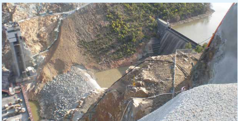
New Cotter Dam (under construction) and old Cotter Dam
