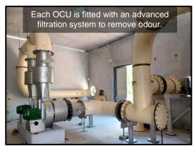
The OCUs have been designed to improve the ventilation of the Belconnen trunk sewer, whilst reducing the impact of the existing ventilation system to the community by treating the air through carbon media to remove odour before being discharged.
