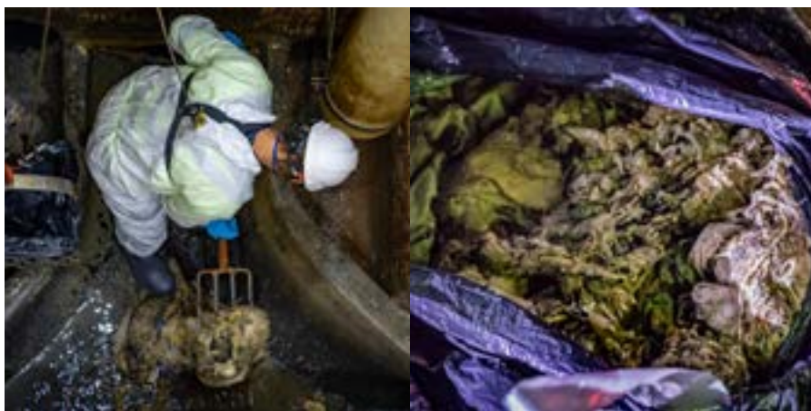
Icon Water worker removing blockage by hand
