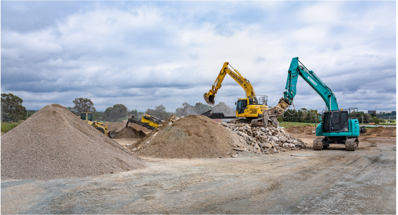
Concrete recycling at Fyshwick Material Storage Area.
